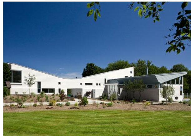
Figure 12 – Butterfly Roof System. Note: 1290 Live/Work Residence designed by Sigrid Miller Pollin. Retrieved January 17, 2013, from http://millerpollin.com/a-and-p/singlefamily/1290/1290.html#
