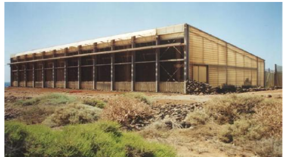
Figure 9 – Seawater Greenhouse after construction. Note: The Seawater Greenhouse. (2010). Retrieved January 17, 2013, from http://myhero.com/go/hero.asp?hero=Seawater_Greenhouse
